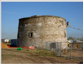
Example: Martello Tower, Essex, UK
